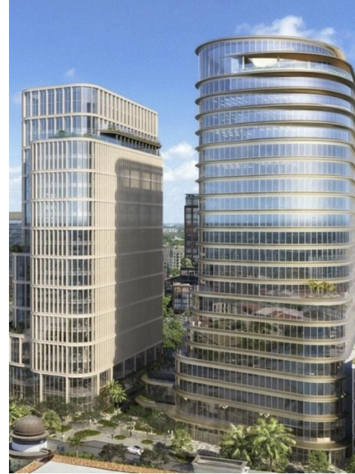
10 & 15 CityPlace Break Ground in West Palm Beach, Delivering Close to 1 Million Office SF - Floridian Development
